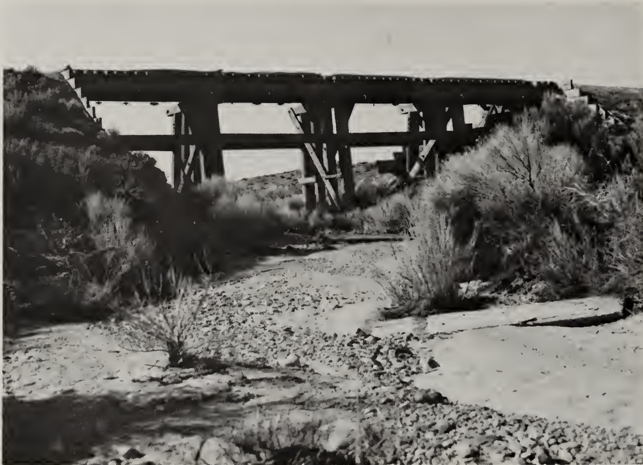
Figure 93: Trestle-work bridge over Rosebud Creek (BLM photo)
